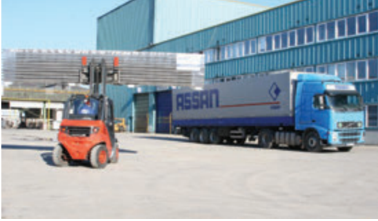
Assan Panel - Tuzla Facilities
